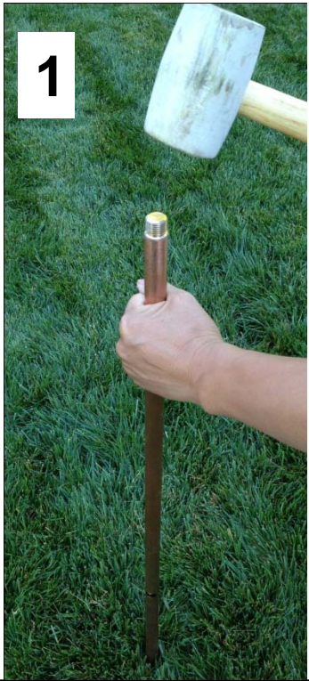
Hammer the main pole into the ground using a Rubber Mallet until the black line touches the ground (about 1 ft deep).
